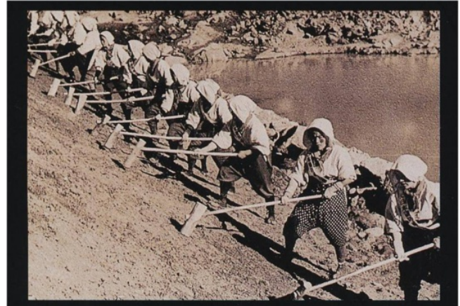
Fig. 6. A traditional construction technique of compacting soil for reservoirs in Japan.
