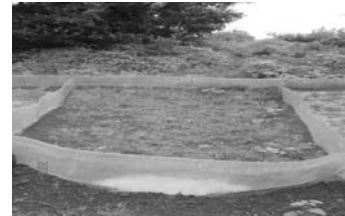
Fig. 6. Plot without Geotextile.
