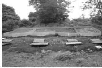
Fig. 2. View of plots After Installation of Geotextile.
