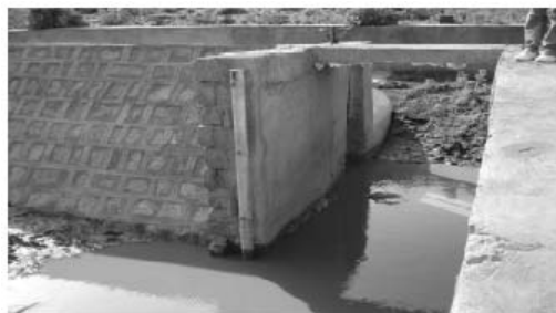
Fig. 3. Pressure gauge installed at intake point.
