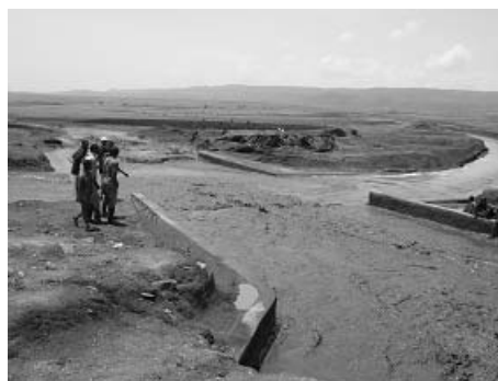
Fig. 3. Flood over the hydraulically regulated structure.
