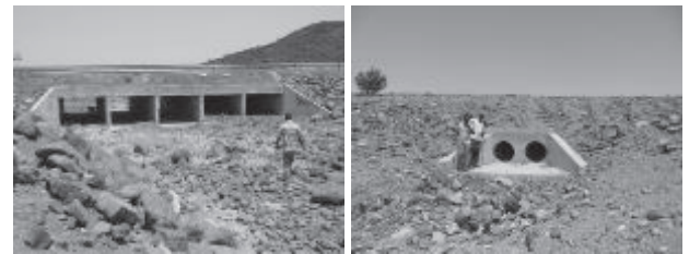
Fig. 7. Concrete culvert crossing the main road. Box culvert on left and pipe culvert on right.
