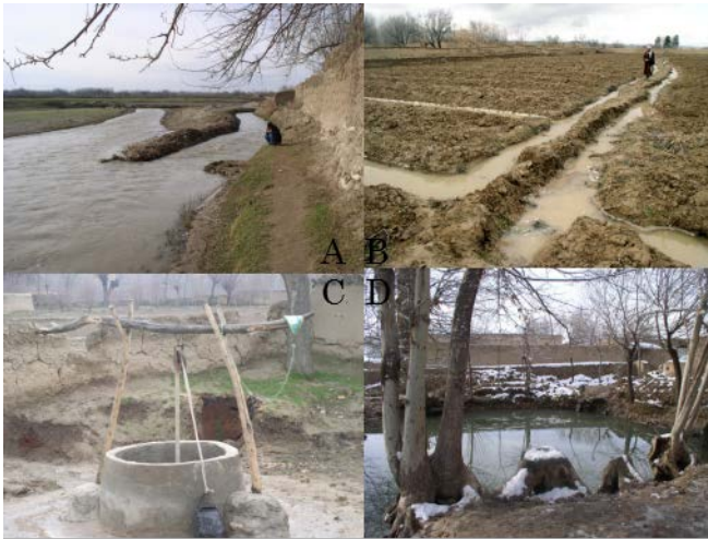
Fig. 6. Typical irrigation facilities in Afghanistan. A: intake gate in river, B: earth canals, C: shallow well, D: irrigation pond
